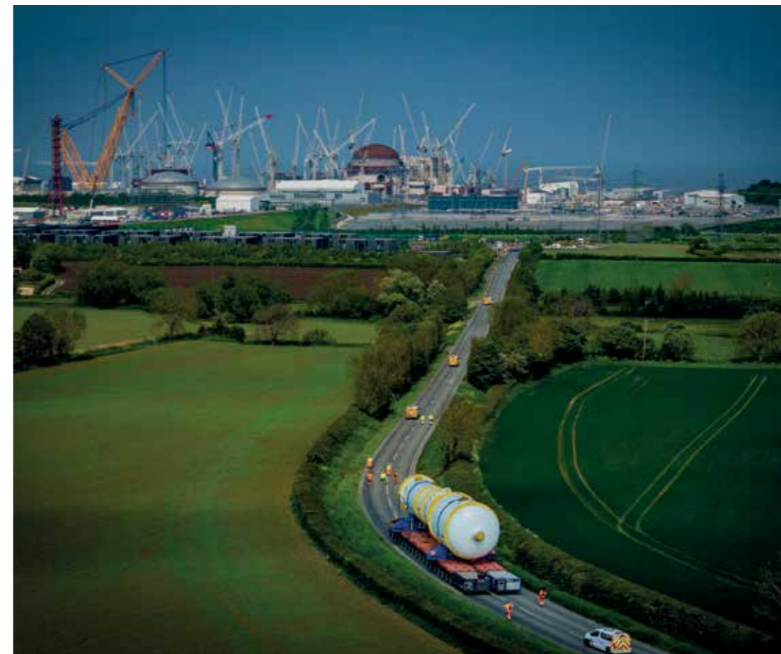
Above: HPCs eight steam generators will drive the two giant Arabelle turbines at the plant
